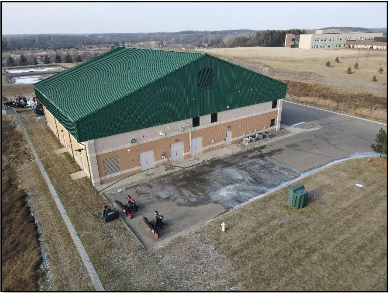
Water Treatment Facility
